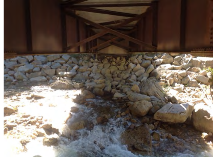
Left Bank Abutment when facing downstream
