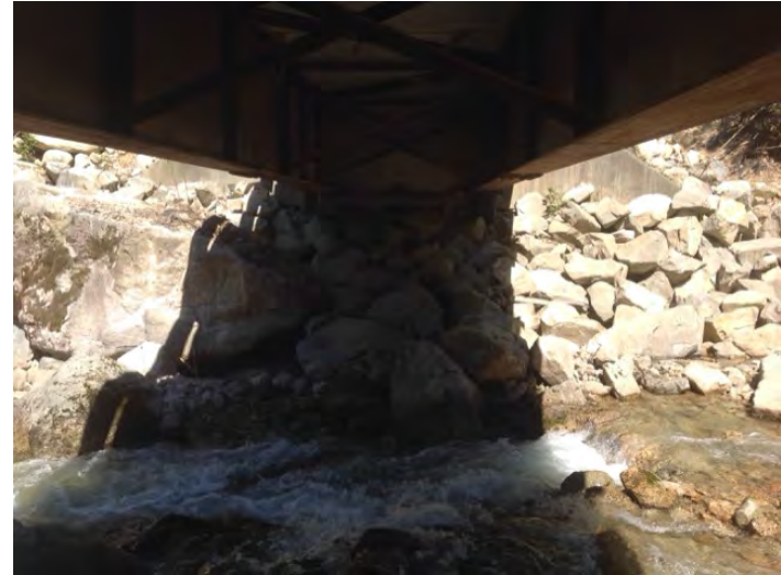
Right Bank Abutment when facing downstream
